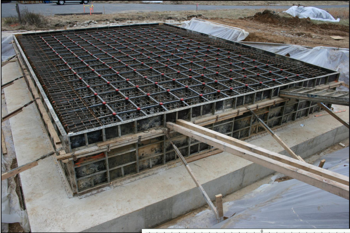
Above: Seismic mass with anchor frame and 192 anchors M24.
